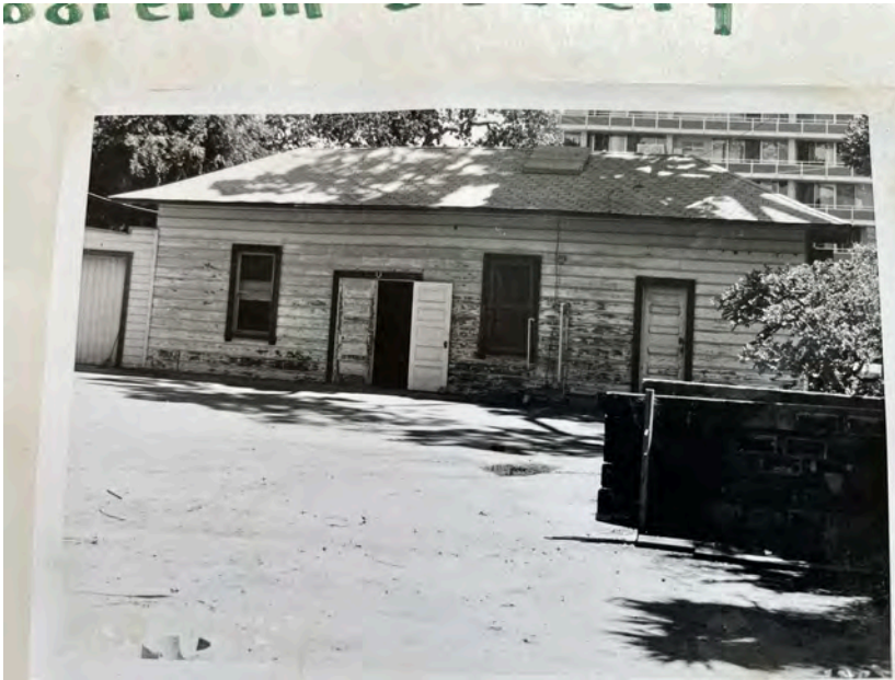
The back of pump-house prior to refurbishment
