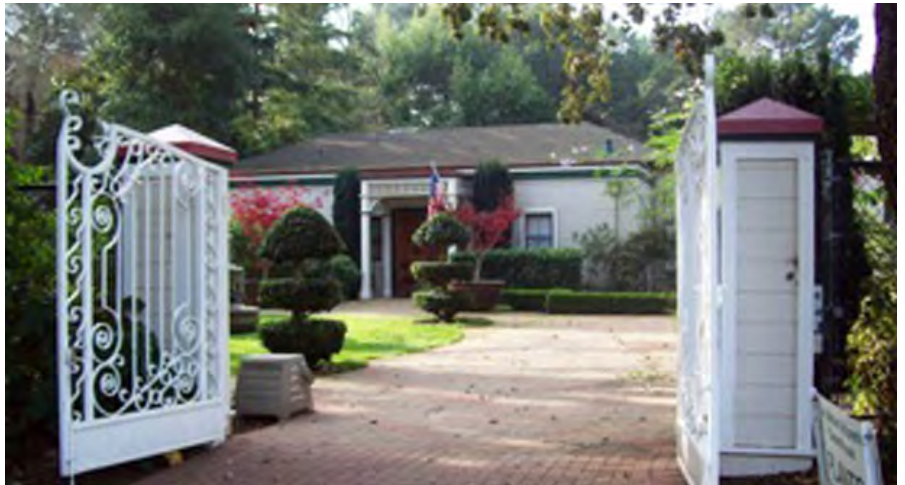
The front of the pump-house today
